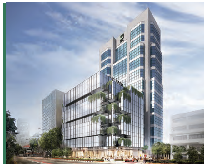
Both Odeon Towers and its extended building were awarded Green Mark Platinum certification.
