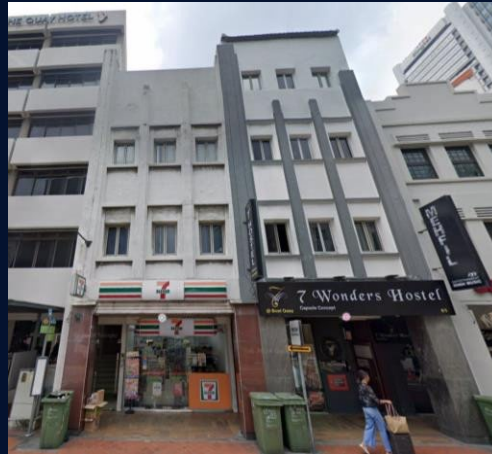
63 & 65 South Bridge Road
