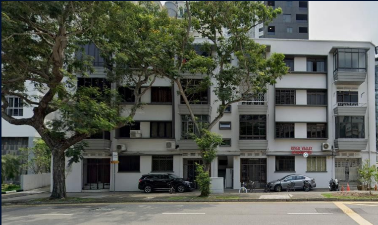
River Valley Apartments
