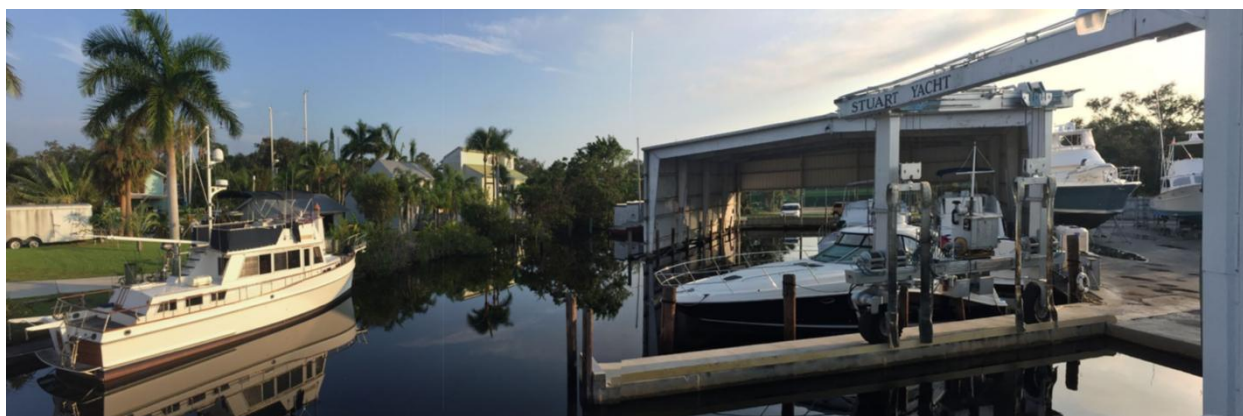
Photo of Stuart Service Yard located at 450, SW Salerno Road Stuart, Martin County, Florida, U.S.
