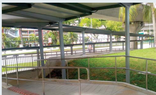
OKP is involved in infrastructure works under the Walk2Ride programme, such as covered linkway to new ramp at South View LRT.
