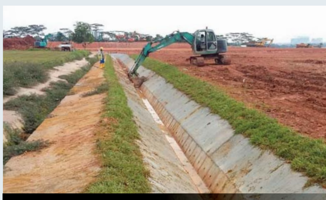
OKP is involved in the construction of road and drains at North Coast Avenue, trunk sewer at Admiralty Road West and North Coast Avenue and junction improvement at Attap Valley Road.
