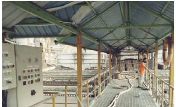
Staff monitoring water condition at the water treatment plant
