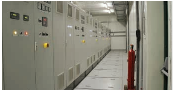
The control room
