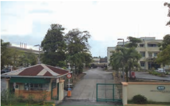
The office and factory in Ijok, Malaysia
