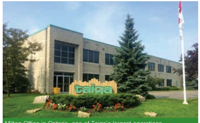
Milton Office in Ontario, one of Taiga's largest operations
