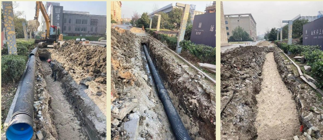
Excavation and replacement works of drainage pipes in the Beigang facility
