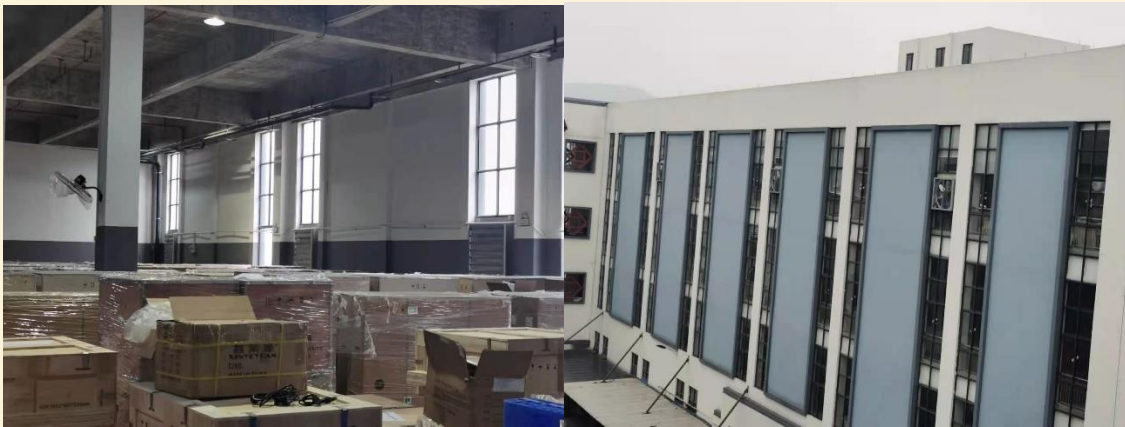
An interior and exterior look at the installed ventilation fans
