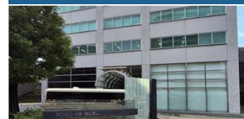
Toyo MK Fuso Building
