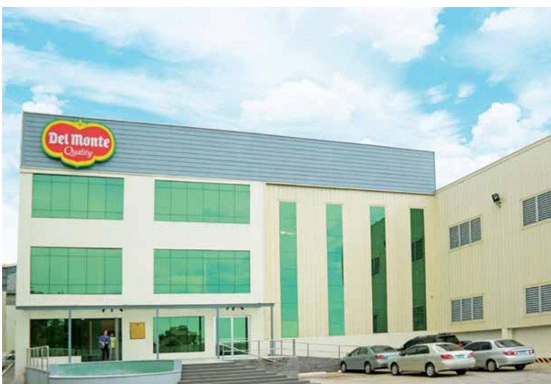
New in-house PET plant in the Philippines
