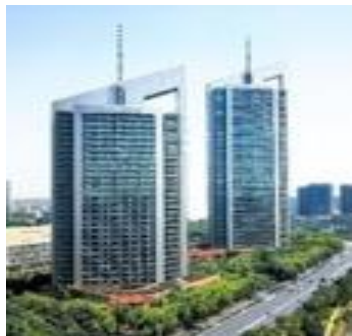
Yanlord International Apartments, Tower A, Nanjing (Closed down for renovation) 仁恒国际公寓, A栋, 南京
