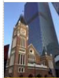
Office Tower on the Old Treasury Building site
