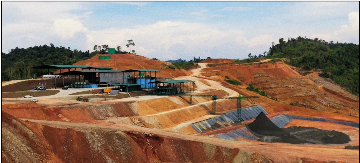
Figure 3.6 Sokor CIL plant and tailings facility – January 2018
