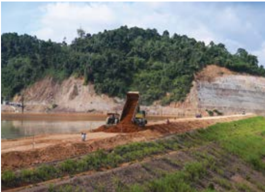
Raising of tailing dam
