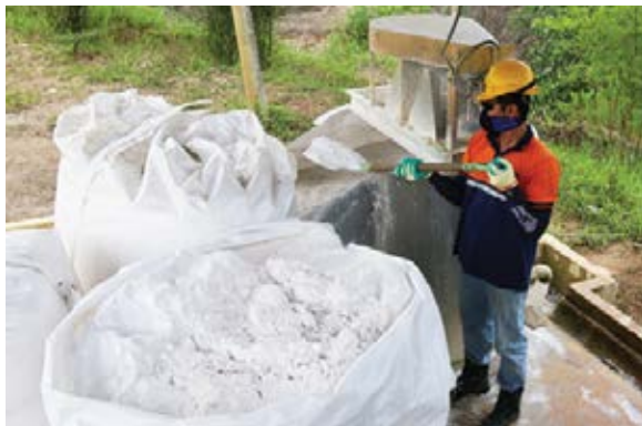
Mine effluent treatment using hydrated lime
