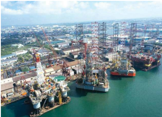
Keppel FELS, Singapore
