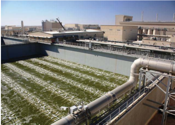
Doha North Sewage Treatment Works, Qatar
