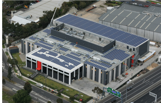
SEEK uses NEXTDC M1 Melbourne data centre which has a 400kW solar rooftop array.
