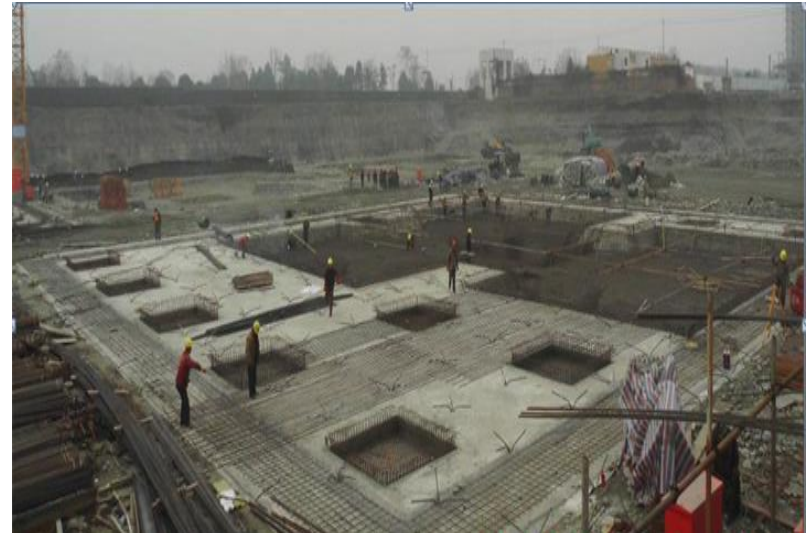
Ongoing construction at a residential block
