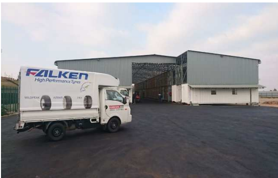
New container warehouse in Johannesburg, South Africa
