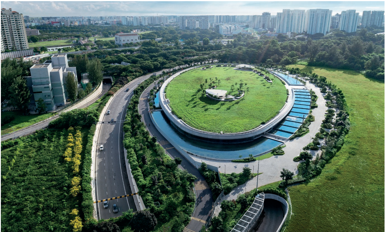
KMEDP is Singapore's only large-scale, dual-mode plant which can treat both seawater and reservoir water.
