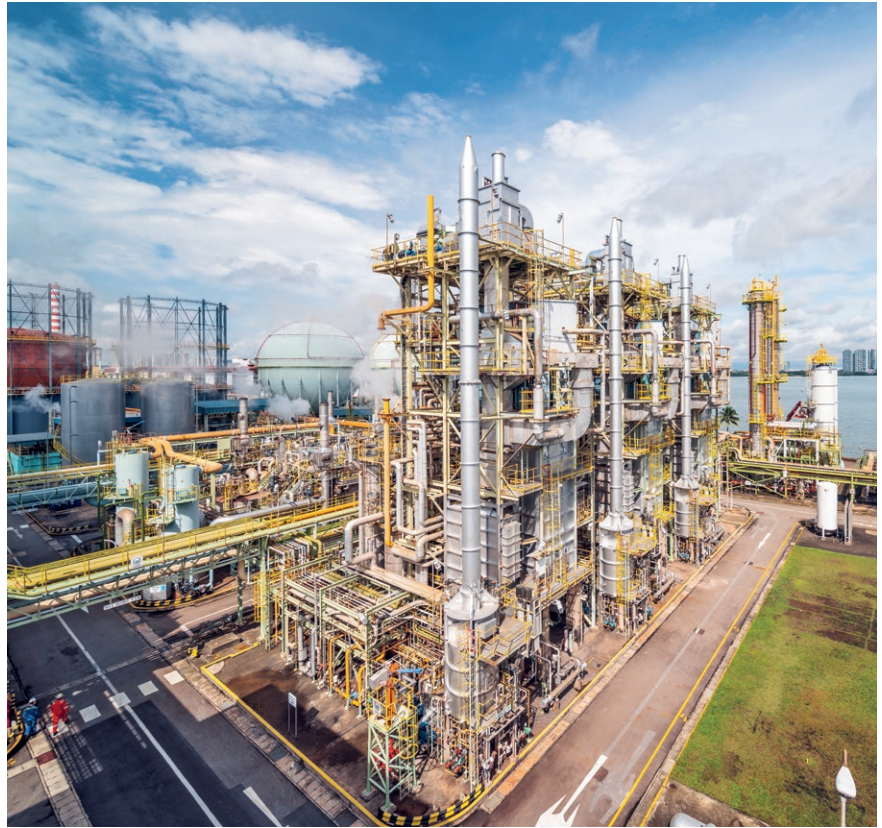
Town gas is produced by City Energy at Senoko Gasworks, Singapore's only town gas plant, with a production capacity of 1.6 million m 3 per day.
