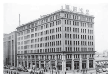
Former head office building
