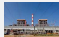
TPCIL Unit 1, India 660 MW
