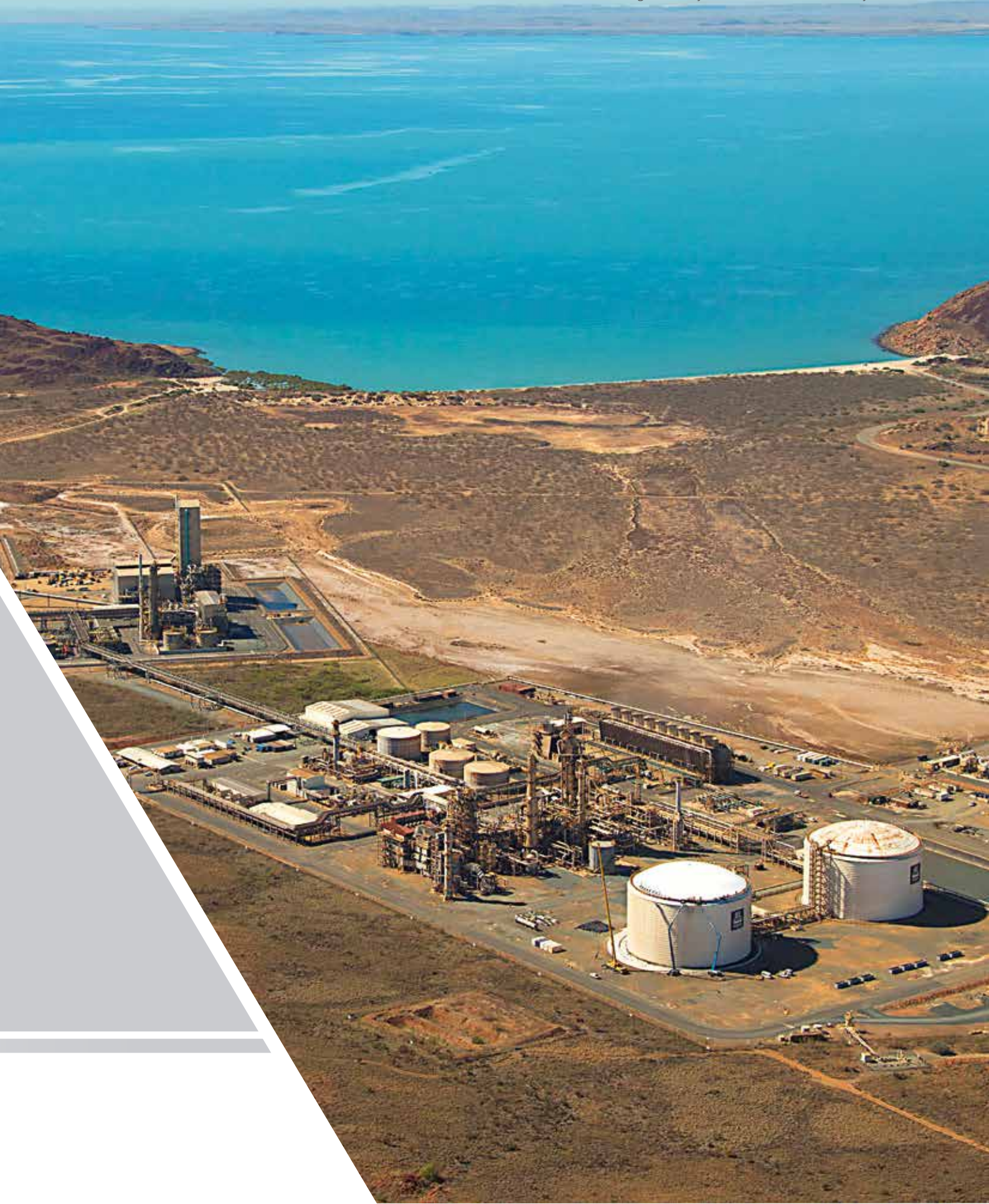
Yara Pilbara Ammonia Plant, Burrup Peninsula, Western Australia. Image courtesy of Yara Pilbara Fertilisers Pty Ltd.
