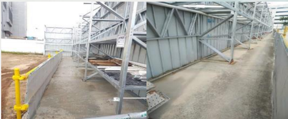
Clean & Unobstructed Site Access/Entry
