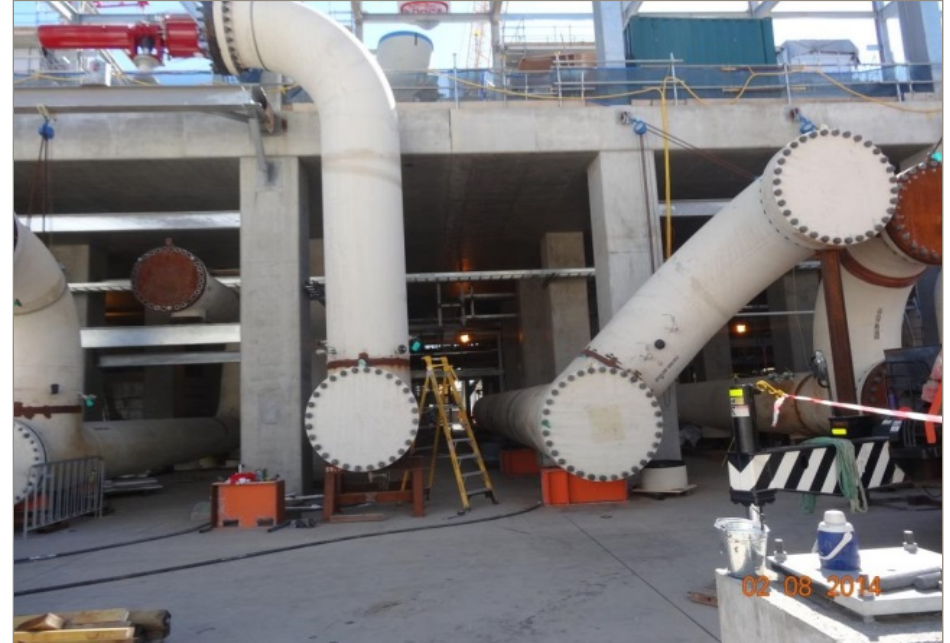
Large-Bore Spools Ready for Pneumatic Testing
