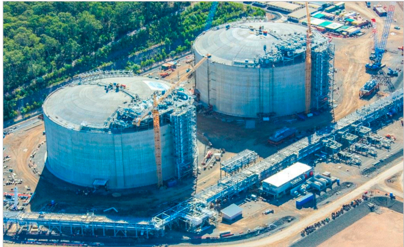
Hydro testing complete on both LNG Tanks
