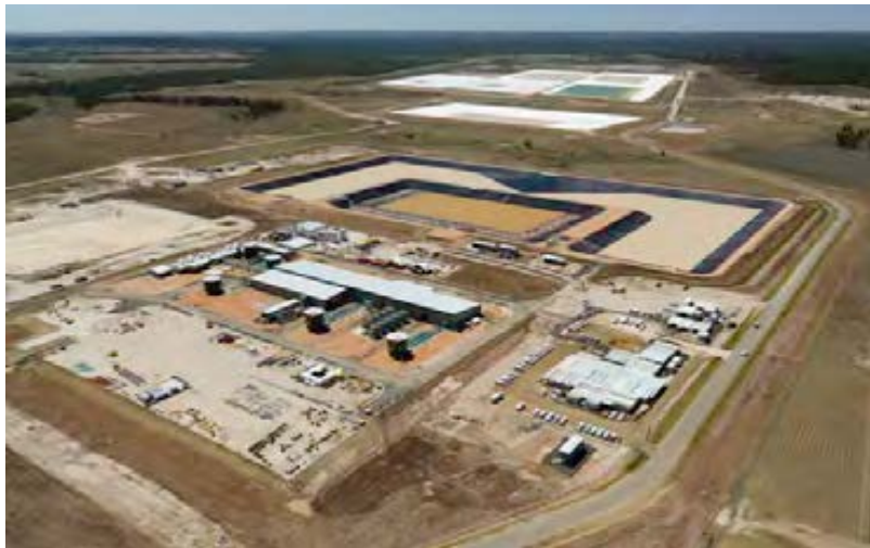
Reedy Creek – water processing facility, October 2014
