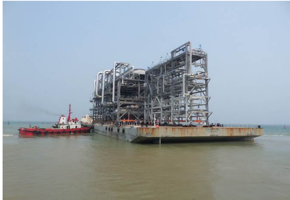
Cryo/AGRU Rack (202DB) & Methane/NRU Cold Box Rack (202GA) Sailed away 6 October 2014
