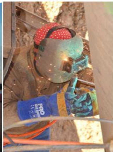
Last Golden Weld on the Main Transmission Pipeline
