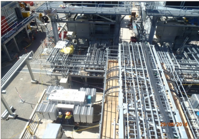
Pipe and Cable Installation Progressing
