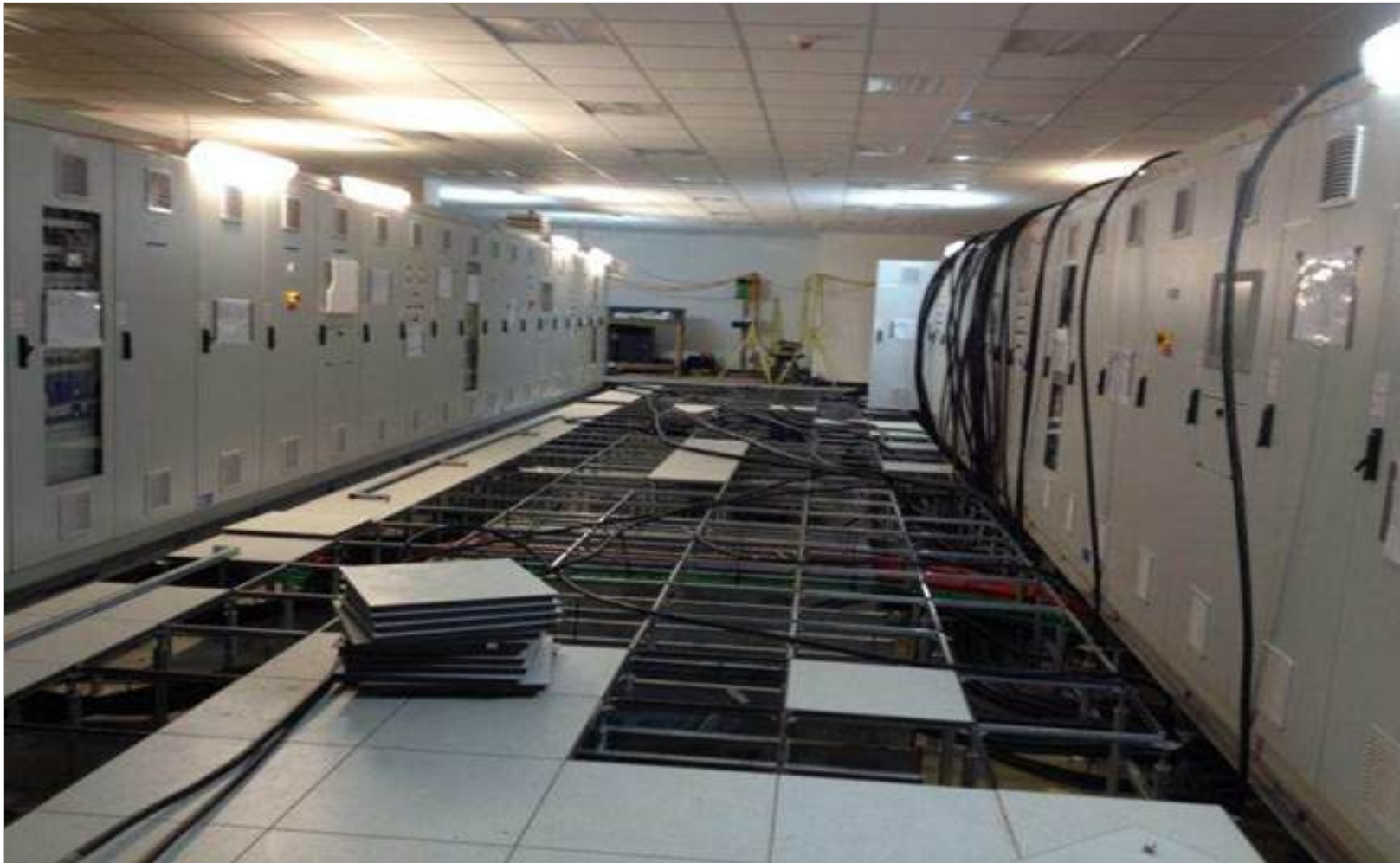
Train 1 Compressor Control Building, Cable Pulling under Floor
