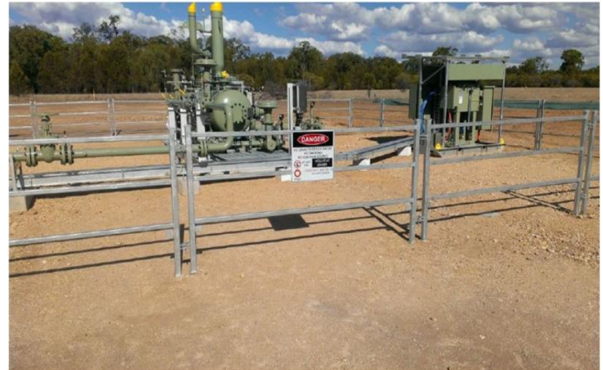
Orana completed Wellhead Separator Installation
