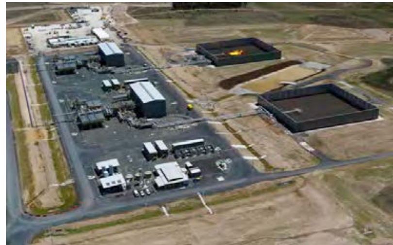
Orana – gas processing facility, October 2014
