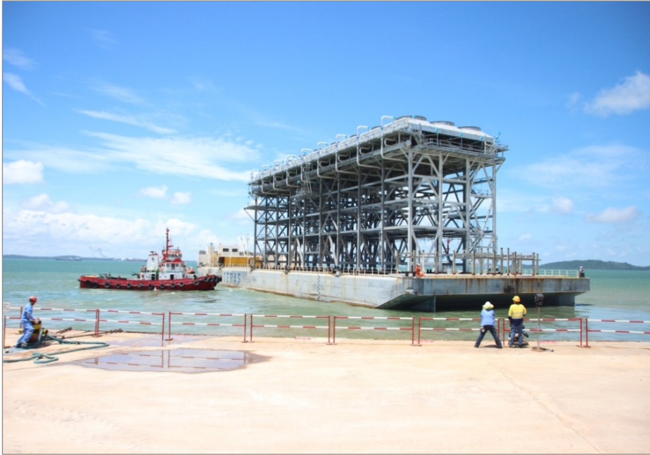
Shipment of Propane Condenser Module 202NA – 9 August
