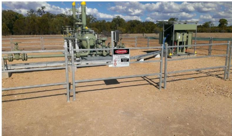
Orana completed Wellhead Separator Installation
