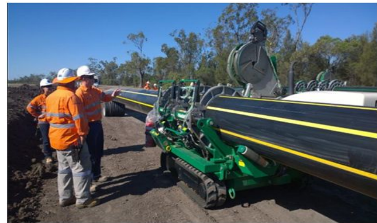
First Weld at Seven Trees Reedy Creek
