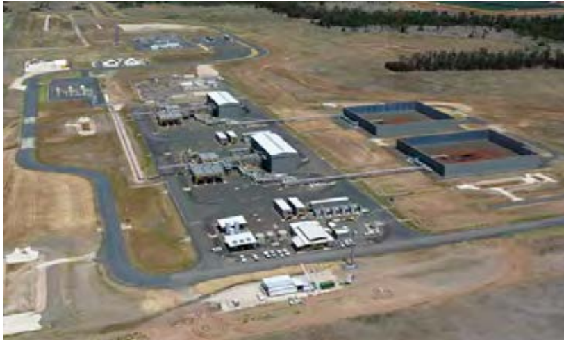
Condabri Central – gas processing facility, October 2014
