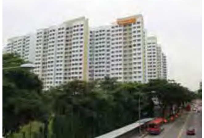
HDB Paya Lebar Road
