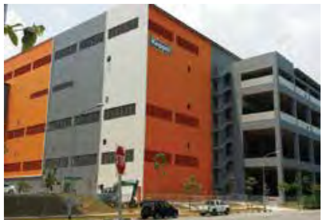
Keppel Logistics @ Greenwich Drive
