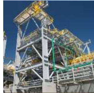
STRUCTURAL MECHANICAL & PIPING INSTALLATION
