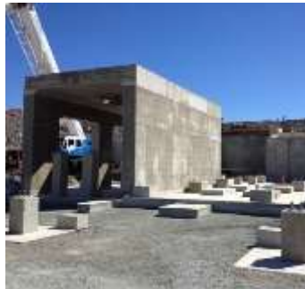
SITE CIVIL WORKS
