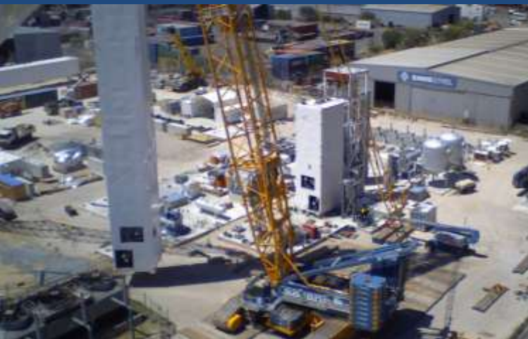
Below: Civmec's multi disciplinary team at delivering site civil works, fabrication and SMP works for BOC's Kwinana Gas Plant upgrade.
