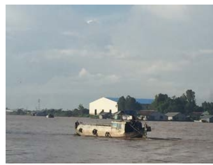
View of IEVNV Biomass plant from the river
