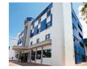
511/513 Yishun Industrial Park A
