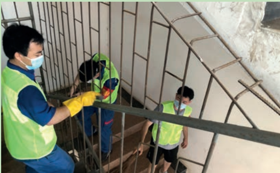
Volunteers helped to renovate the stair handrails, gates and other public facilities of the village committee office building in Nabo Village
