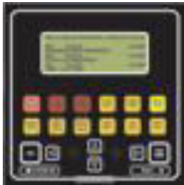
Fire Alarm System
