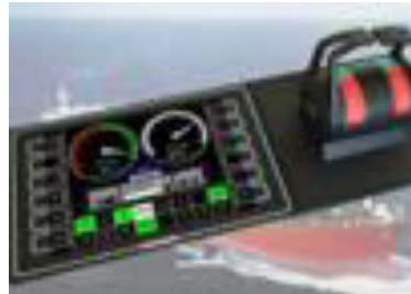
Propulsion Control System
