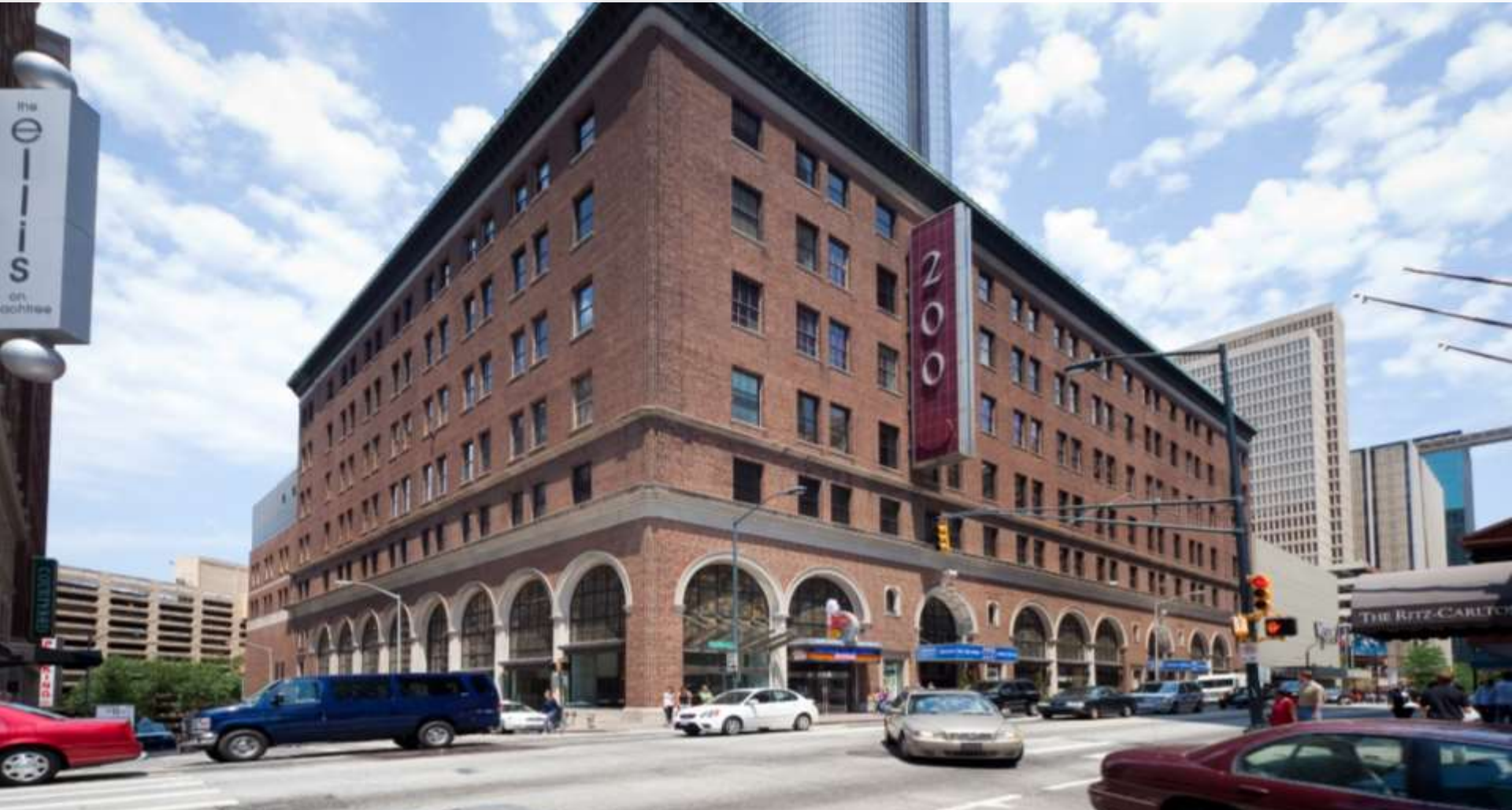
Hi-Tech Building, 180 Peachtree, Atlanta
