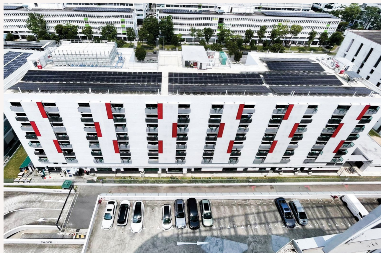
Solar panels at Westlite Ubi
