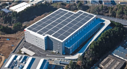
1 ESR Sakura Distribution Centre
