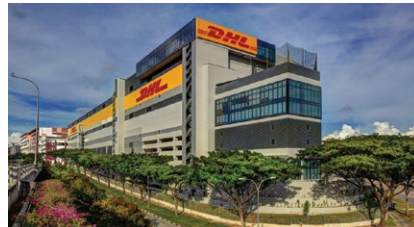
5 1 Greenwich Drive (DHL Supply Chain Advanced Regional Centre)
