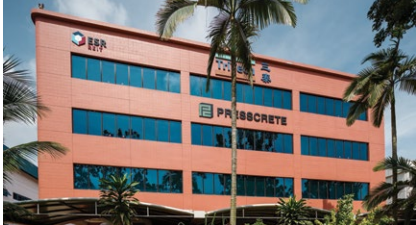
2 31 Changi South Avenue 2
