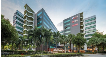
3 2, 4, 6 & 8 Changi Business Park Avenue 1 (ESR BizPark @ Changi)
