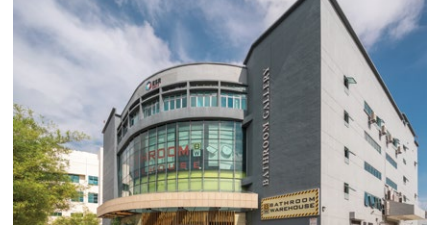
3 25 Changi South Avenue 2
