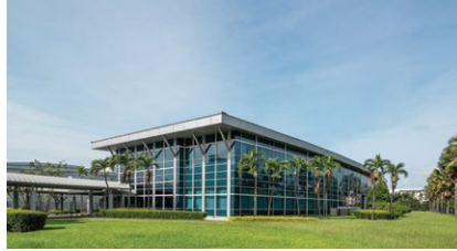
17 3 Tuas South Avenue 4
