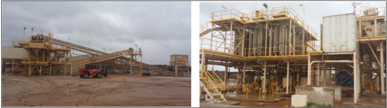
Figure 15: Photos of processing plant at Bald Hill.
