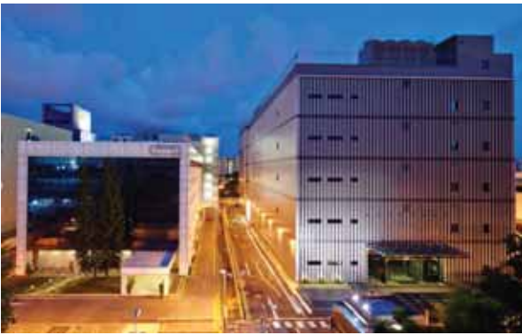
Keppel Datahub 2 (right)
