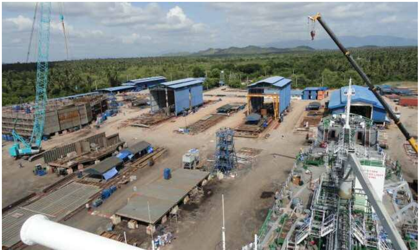
Above: Our shipyard in Thapsakae, Thailand, with 70,000 sqm of land space to undertake EPC projects and provide new building services such as offshore modules and oil rigs structures. We have successfully completed two EPC projects in this shipyard, and have successfully launched and delivered them to our customers.
