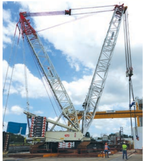
Location: Singapore Equipment: 600 Ton Crawler Crane, 500 Ton Mobile Crane Scope of Work: Heavy Lifting Services
