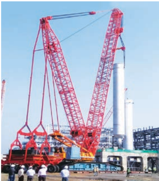
Location: India Equipment: 300/550/1250 Ton Crawler Cranes Scope of Work: Heavy Lifting Services
