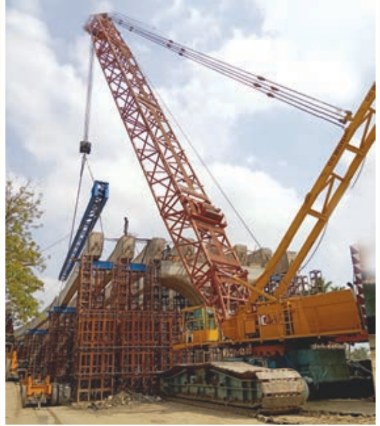
Location: India Equipment: 550 Ton Crawler Crane Scope of Work: Equipment Rental
