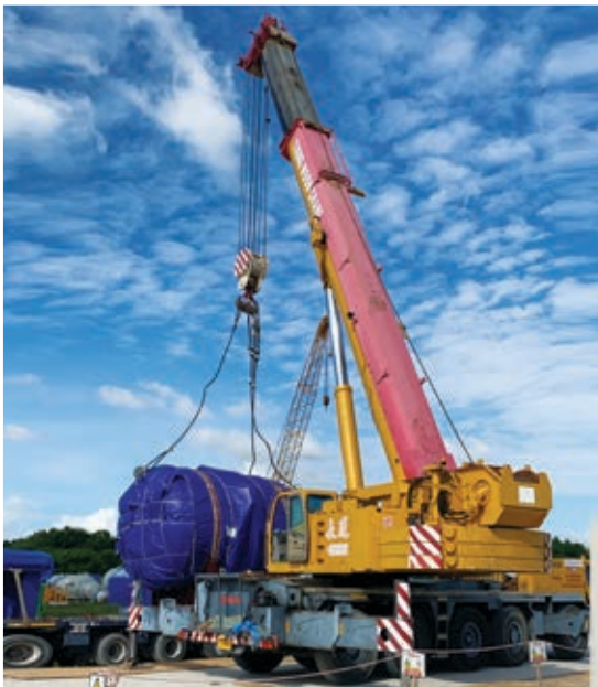
Location: Thailand Equipment: 120 Ton Mobile Crane Scope of Work: Heavy Lifting Services
