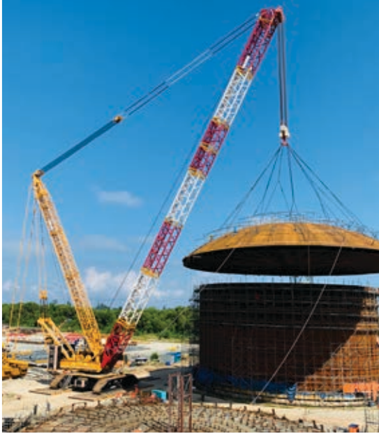
Location: Brunei Equipment: 150/250/280/600/1250/1600 Ton Crawler Cranes, 30/50/60/100/120 Ton Mobile Cranes, SPMT Scope of Work: Heavy Lifting and Transportation Services
