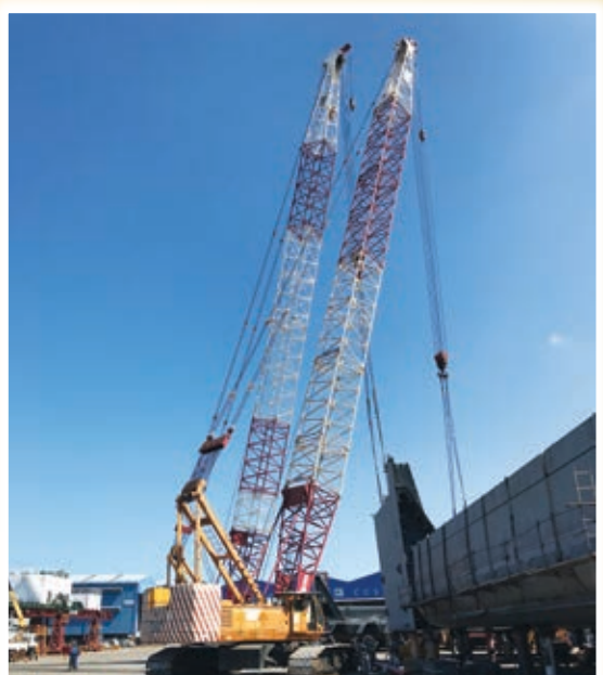
Location: Vietnam Equipment: 280 Ton Crawler Crane Scope of Work: Equipment Rental
