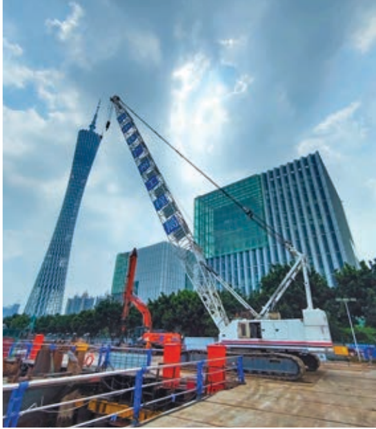
Location: China Equipment: 120 Ton Crawler Crane Scope of Work: Heavy Lifting Services
