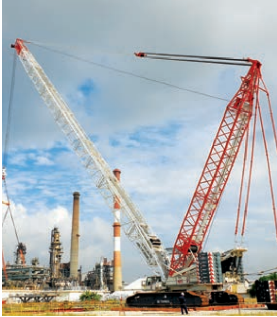
Location : Singapore Equipment : 250/500/600/700 Crawler Cranes Scope of Work : Heavy lifting services
