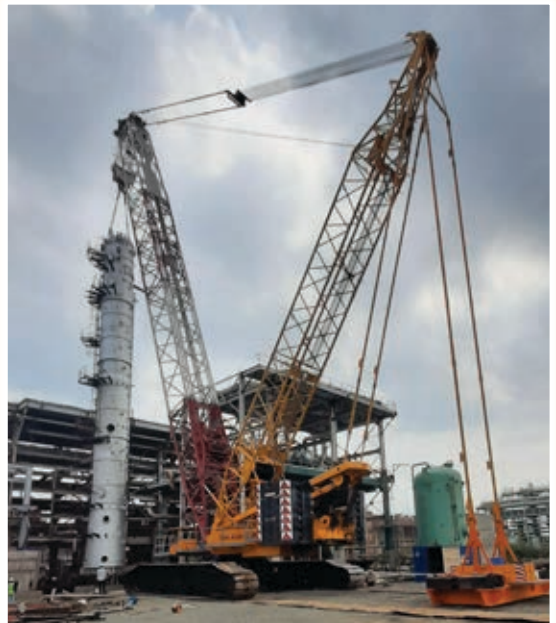
Location: India Equipment: 600 Ton Crawler Crane Scope of Work: Equipment Rental
