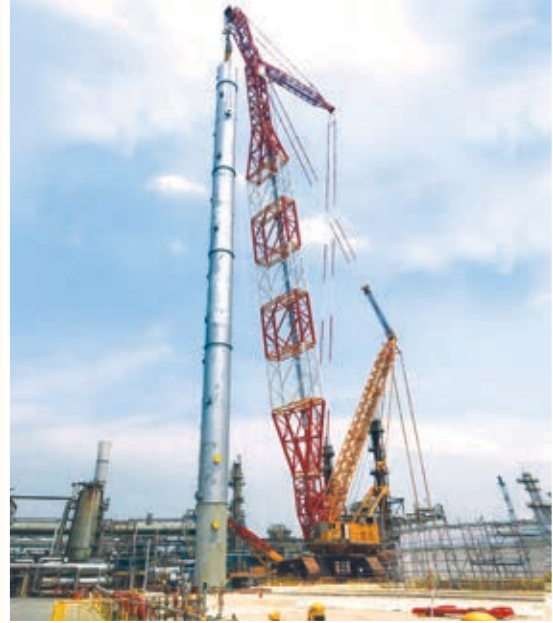
Location: Singapore Equipment: 1600 Ton Crawler Crane Scope of Work: Heavy Lifting Services
