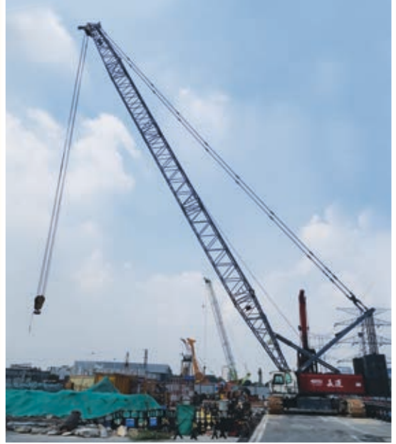
Location: China Equipment: 225 Ton Crawler Crane Scope of Work: Heavy Lifting Services
