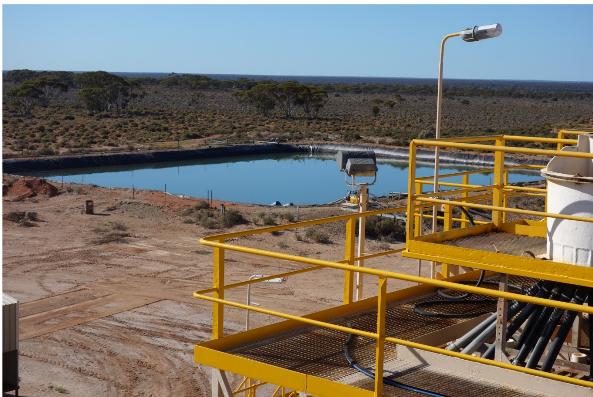
Picture 2: Successful Pre-Commission Testing of the Processing Plant
