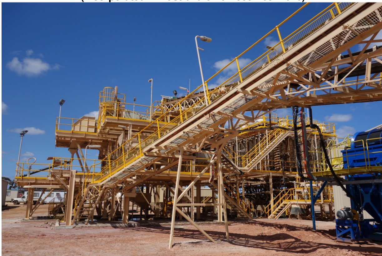
Picture 3: Newly installed Scubber feed system to address the ore from Boreline Pit.
