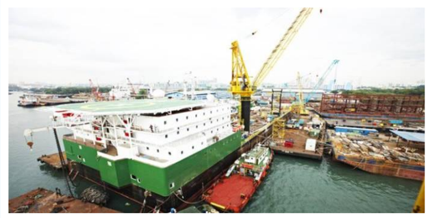
Construction of McDermott LB32 pipelay barge
