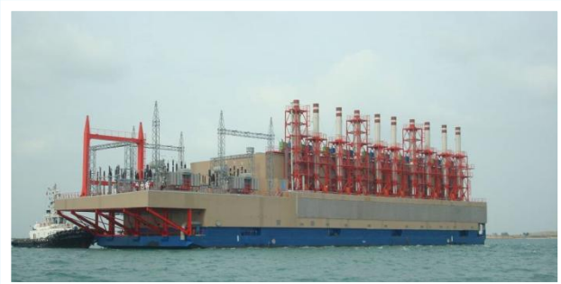
Power Barge Conversion for KPS Alican Bey
