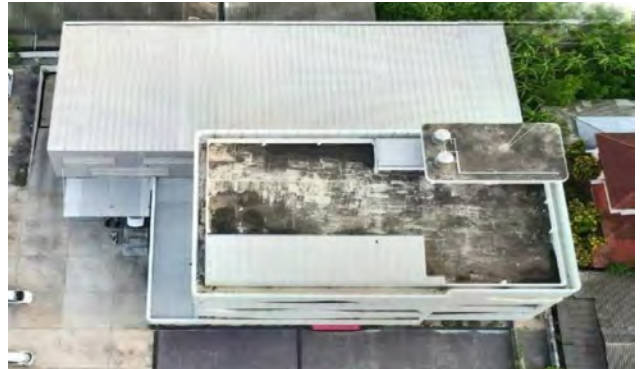
Achieva Digital Thailand Rooftop
