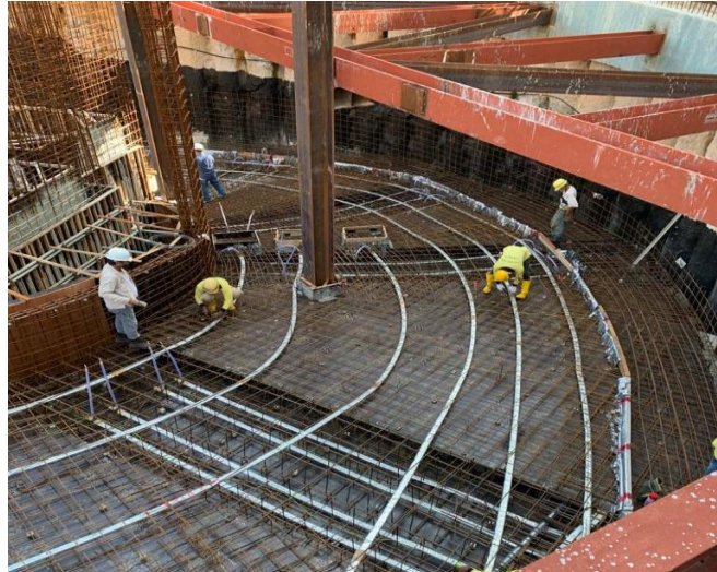
Using post tensioning technology during construction of our project
