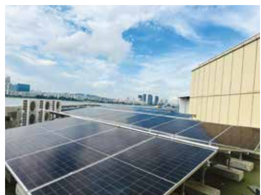
Solar panel installation at 51 Penjuru Road
