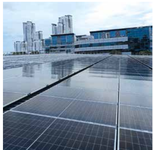
Solar panel installation at 8 Commonwealth Lane
