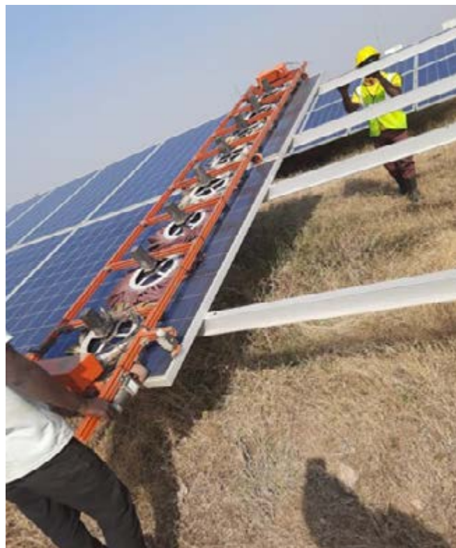
Dry robotic cleaning with microfiber cloth
