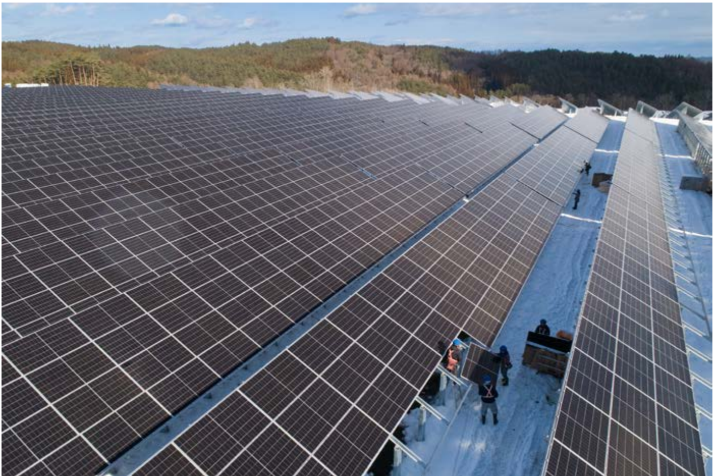
Installation of solar PV panels in Japan
