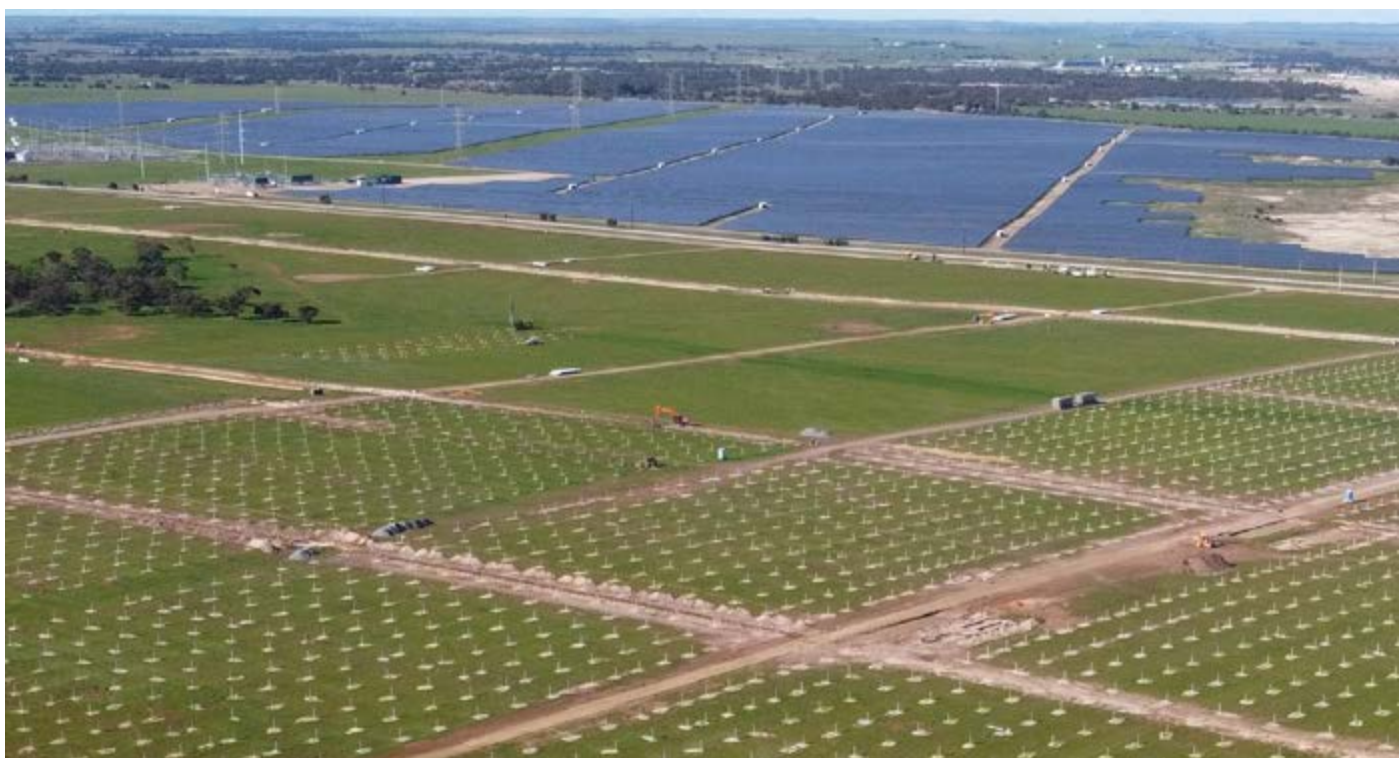
Tailern Bend 2 Project currently under construction in South Australia
