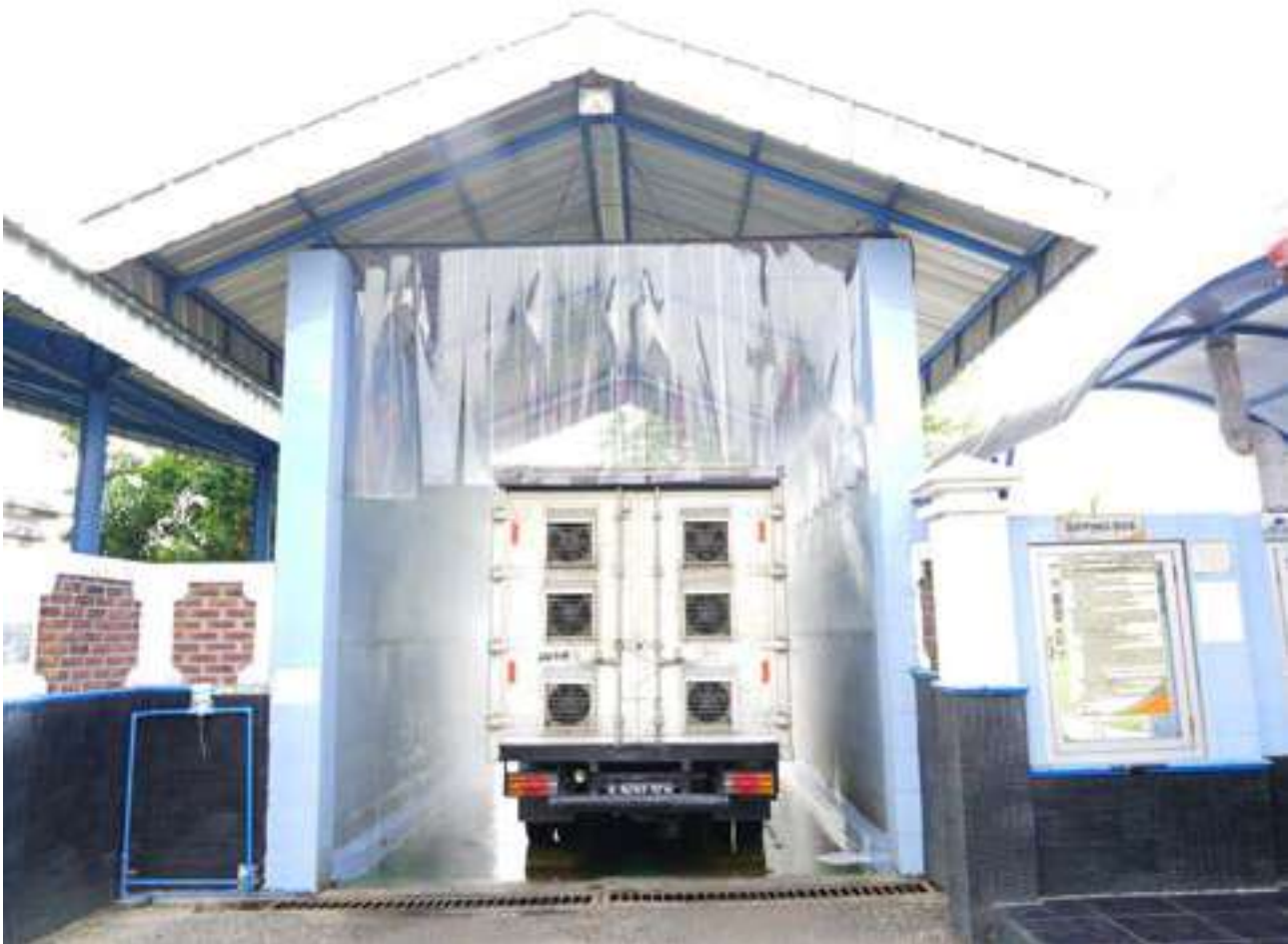
Area Pencucian Kendaraan Vehicle-Washing Area
