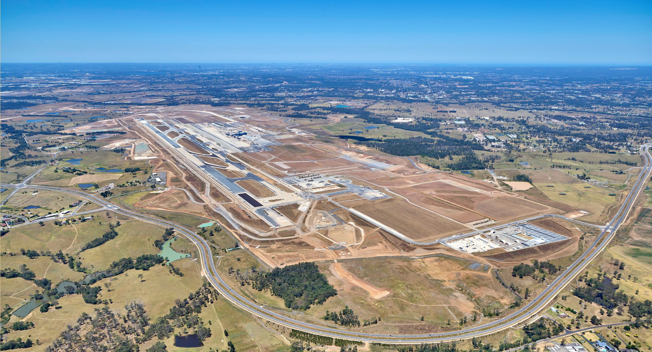
CPB - Western Sydney Airport Airside Civil Earthworks
