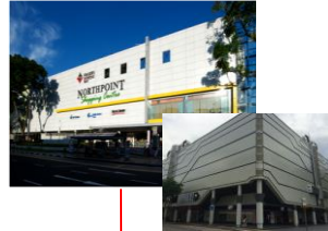
Northpoint City North Wing + Yishun 10 Retail Podium
