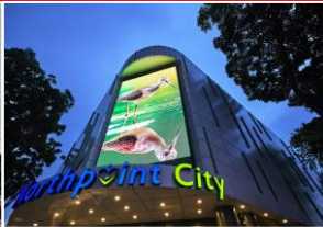
Northpoint City North Wing + Yishun 10 Retail Podium
