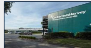
24 41 – 45 Hydrive Close, Dandenong South
