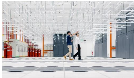
Data hall fit out
