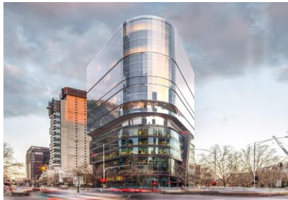
Adina Apartment Hotel Southbank Melbourne
