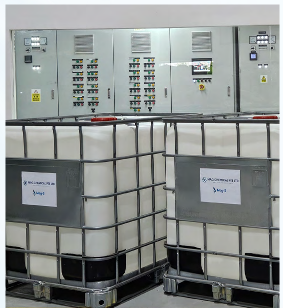
PRODUCTION FACILITIES UNDER MAG CHEMICAL PTE. LTD.
