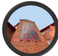
Government infrastructure and workplaces
