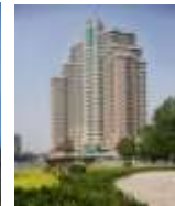
Somerset Olympic Tower Property Tianjin
